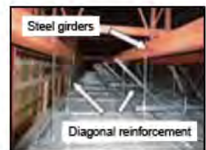
Building renovation using metal-reinforced ceilings
