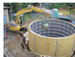
Install a fire cistern
