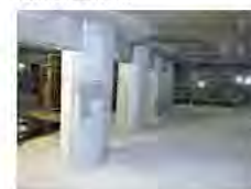
After seismic reinforcement (water purification plant)
