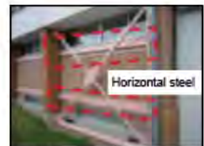
Example of measures to improve the earthquake-proofing of non-structural materials
