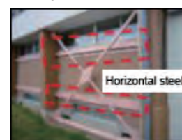
Examples of quake-proofing of non-structural components
