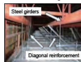
Renovations to metal substrate ceilings
