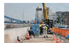
Quake-proofing of coastal levees
