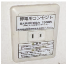
Electrical outlet supplied from solar panel (courtesy of NPO PV-Net)
