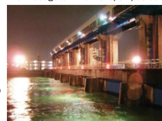
Imai Floodgate closed in preparation for high tides
